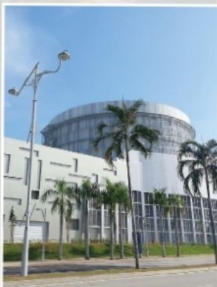
Largest Thermal Storage Tank Insulation & Polyurea Waterproofing
